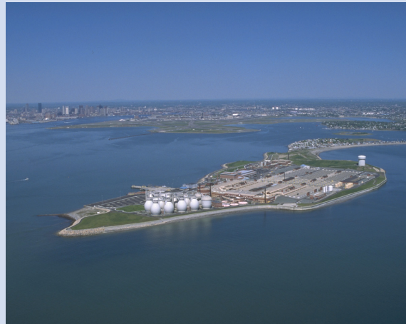
Figure: Deer Island Sewage Treatment Plant. Image courtesy of Massachusetts Water Resources Authority.
