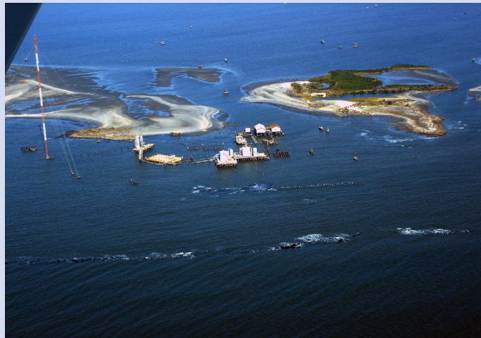
Figure: Aerial photo showing gradual barrier island erosion and subsequent flooding of facilities in coastal Louisiana. Rising sea levels are projected to increase coastal erosion, and the frequency and severity of damaging storm surges and flooding. Image courtesy of Tim Carruthers, Integration and Application Network, University of Maryland Center for Environmental Science ( ian.umces.edu/imagelibrary/ ).
